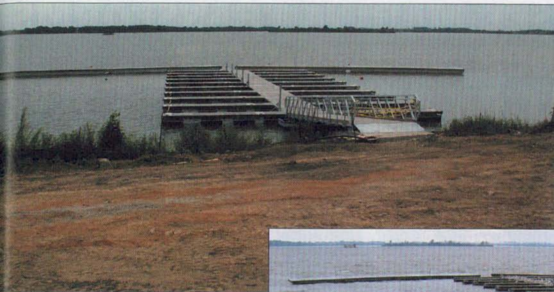
Left: Antigua Cove Marina, one of three deepwater facilities under development at resort community Little Harbor, offers moorage in a Rixö post-tensioned floating concrete dock system.
